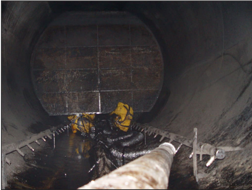
Above: the entry crew is moving past the first of five weir screens inside the vessel to continue removing sludge at the outlet end of the vessel.
