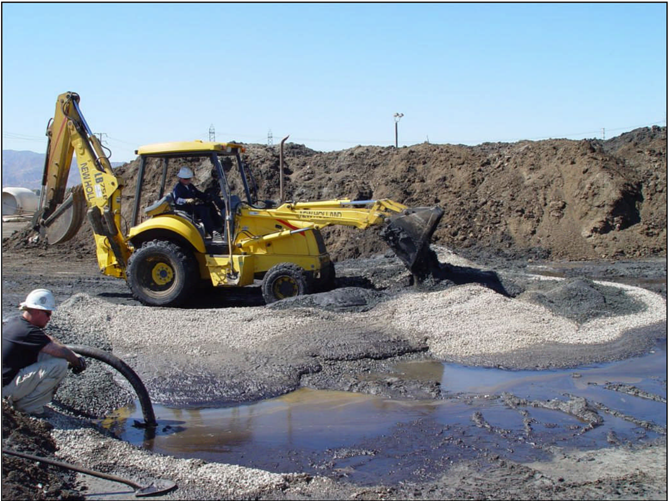
Above: the unloaded fluidized sludge shown in the last slide is shown here being mixed by a skip loader. Below: the load was completely mixed dry and piled in 30 minutes time.
